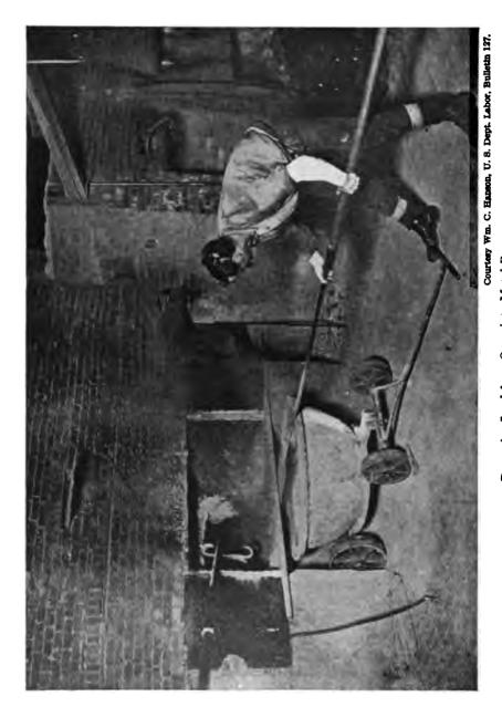
Removing Lead from Oven into Metal Pan.
